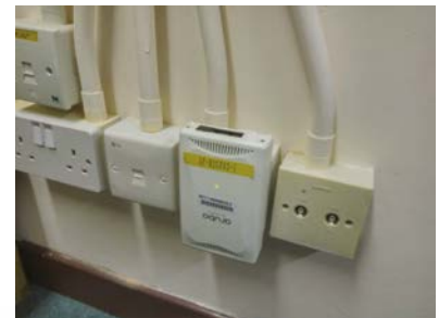
▲ Wi-Fi APs installed in classrooms
