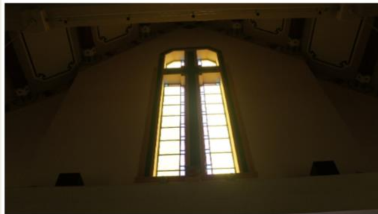
Looking back to the big cross on the main facade from inside. The voids of cross allow light to penetrate into the dark church and created a sense of coming down of god from heaven.
